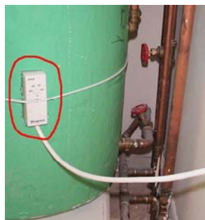
Cylinder Thermostat
