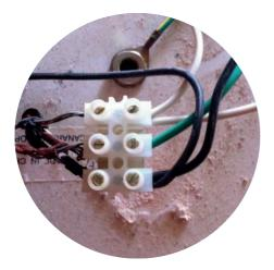
An immediately dangerous situation - Line conductor connected to the metallic enclosure of a light fitting and thermal damage sufficient to permit access to live parts
