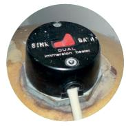
Older immersion heater without thermal cut-out
