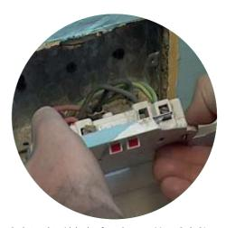
Socket-outlet with broken face plate, requiring a Code C1
