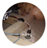
Unsatisfactory connection to a downlighter requiring a Code C2
