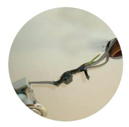
Unsatifactory connection to a downlighter, requiring a Code C2
