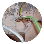
Absence of reliable means of earthing due to inadequate connection
