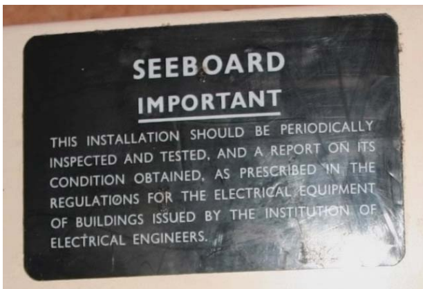
A typical periodic inspection notice for an older installation
