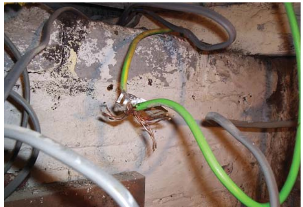
Absence of a reliable means of earthing
