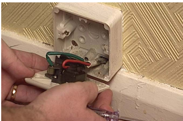
Inspecting a socket-outlet
