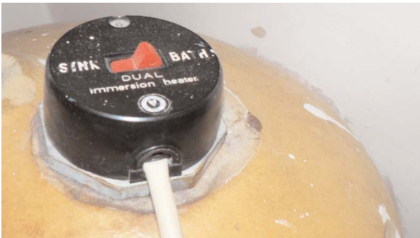
Older immersion heater without thermal cut-out
