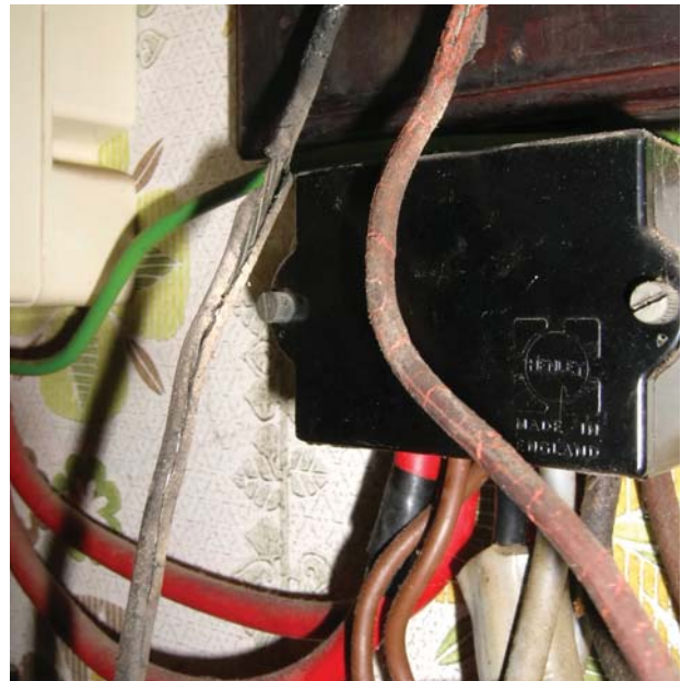
Live parts exposed to touch
