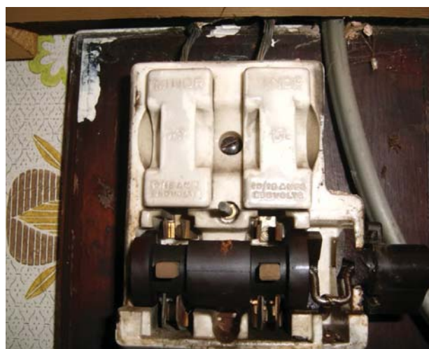
Double-pole switch with fuses in each pole
