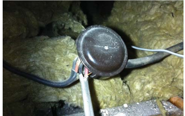
Cable sheaths not taken inside non-conducting enclosure
