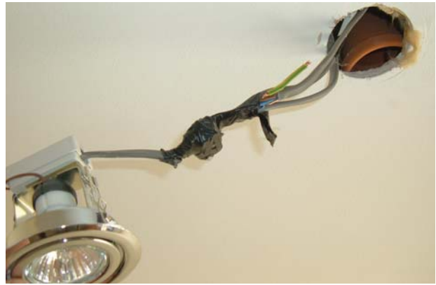
Unsatisfactory connection to a downlighter
