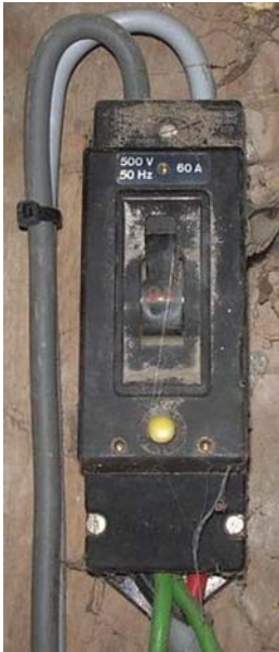
60 A voltage-operated earth-leakage circuit-breaker. (Photo courtesy of RF Lighting)
