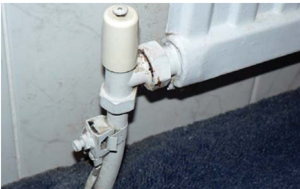
Unmarked bonding conductor
