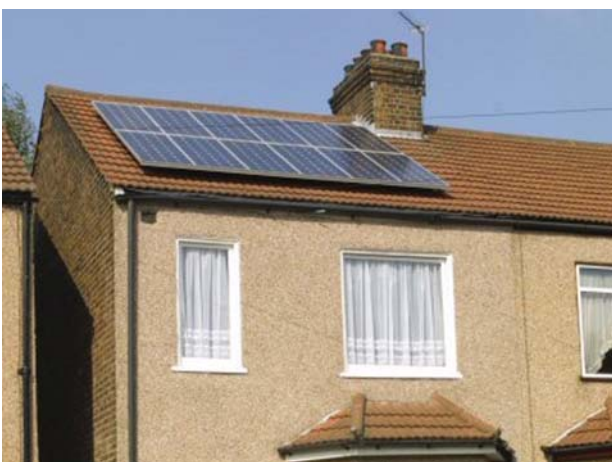
Photovoltaic installation (Photo courtesy Energy Saving Trust)
