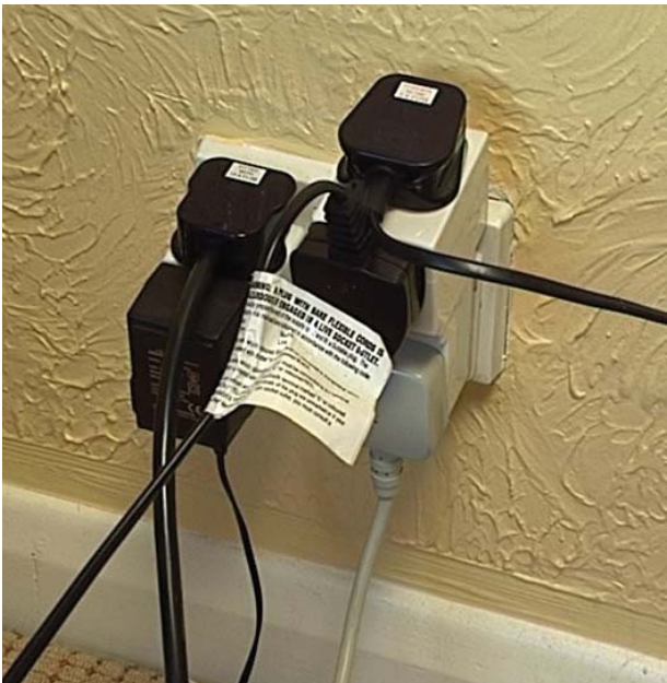
A potentially overloaded socket-outlet
