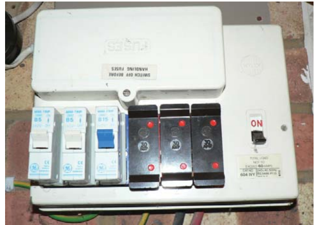
Consumer unit with circuit-breakers and fuses
