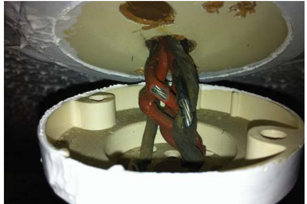
Crumbling vulcanised rubber insulation
