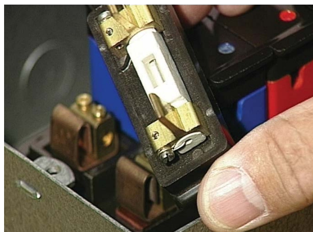
Checking a fuse carrier (base missing)
