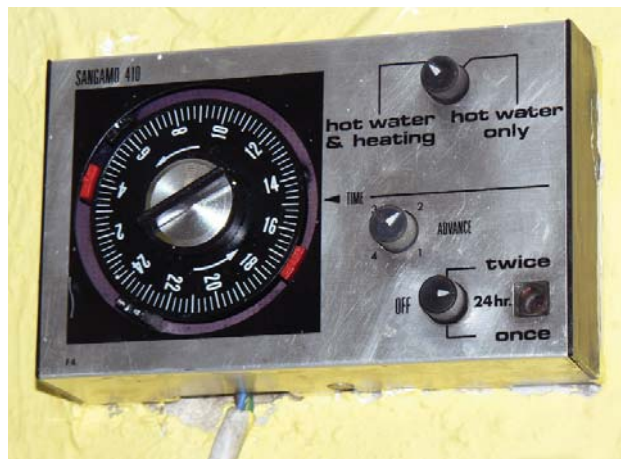
Cable sheath not taken inside metallic enclosure
